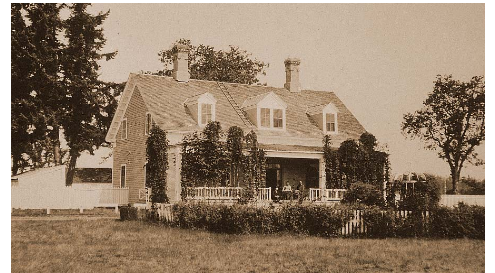
The Commanding Officer's quarters was used as a home for the superintendent of the hospital after the fort was turned over to Washington.
