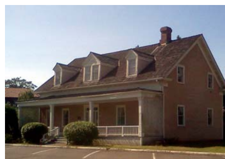
Quarters 2 before and after removal of laurel.
